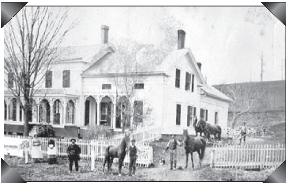
David Hamilton homestead, left wing built in 1815. The property was sold to NY State in 1939 and is now part of Stony Pond State Forest.
