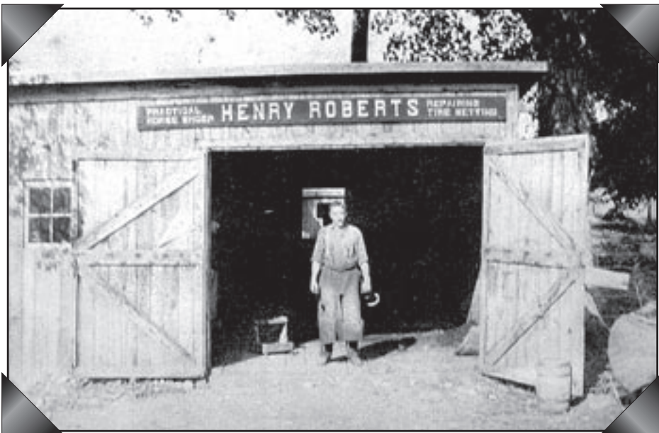
Henry Roberts' blacksmith shop on Cherry Valley Turnpike in Nelson.
