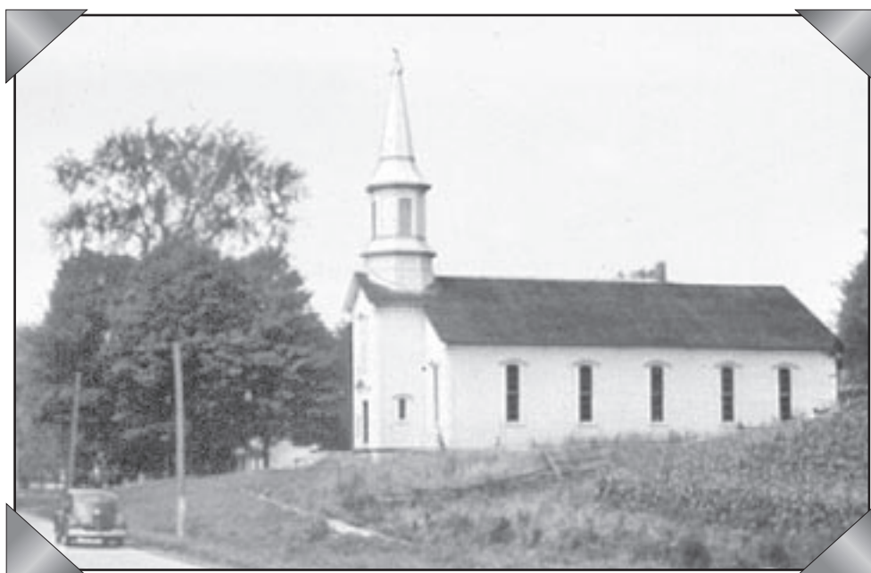
Nelson Methodist Church, Cherry Valley Turnpike 1940
